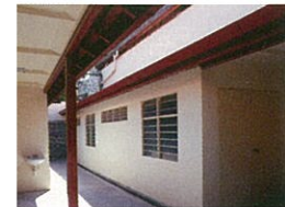
The refurbished back courtyard
