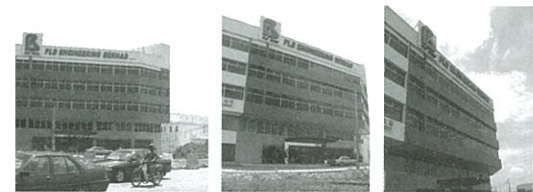
View of the completed project
