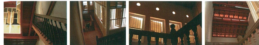
View of staircase from ground floor
