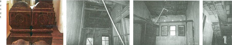
Detail of stair balustrade
