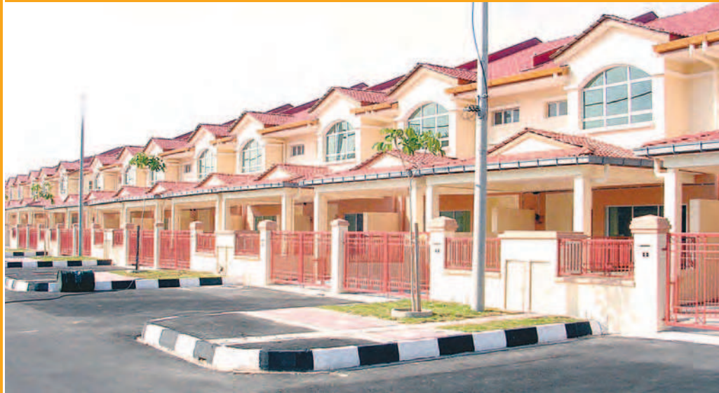
Actual constructed terrace houses.
