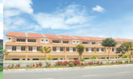
Actual shop offices during construction
