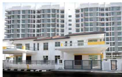
View of both the double storey semi detached units and the apartment block behind
