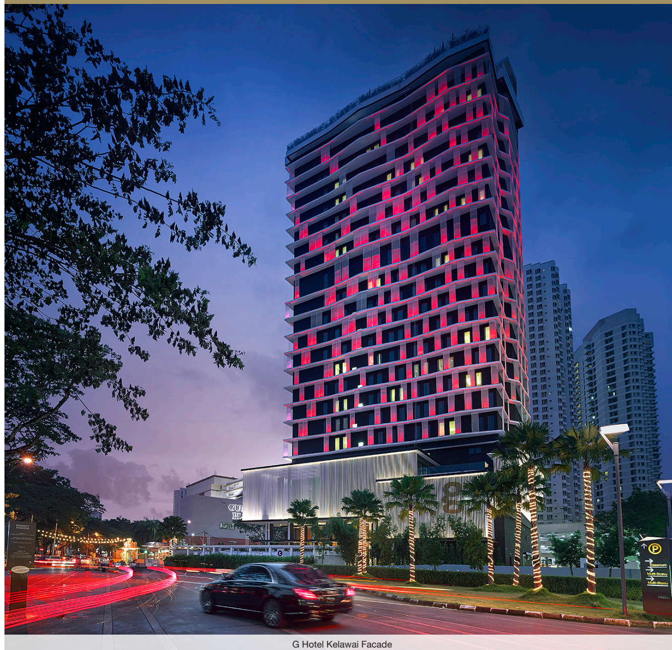
G Hotel Kelawai Facade
